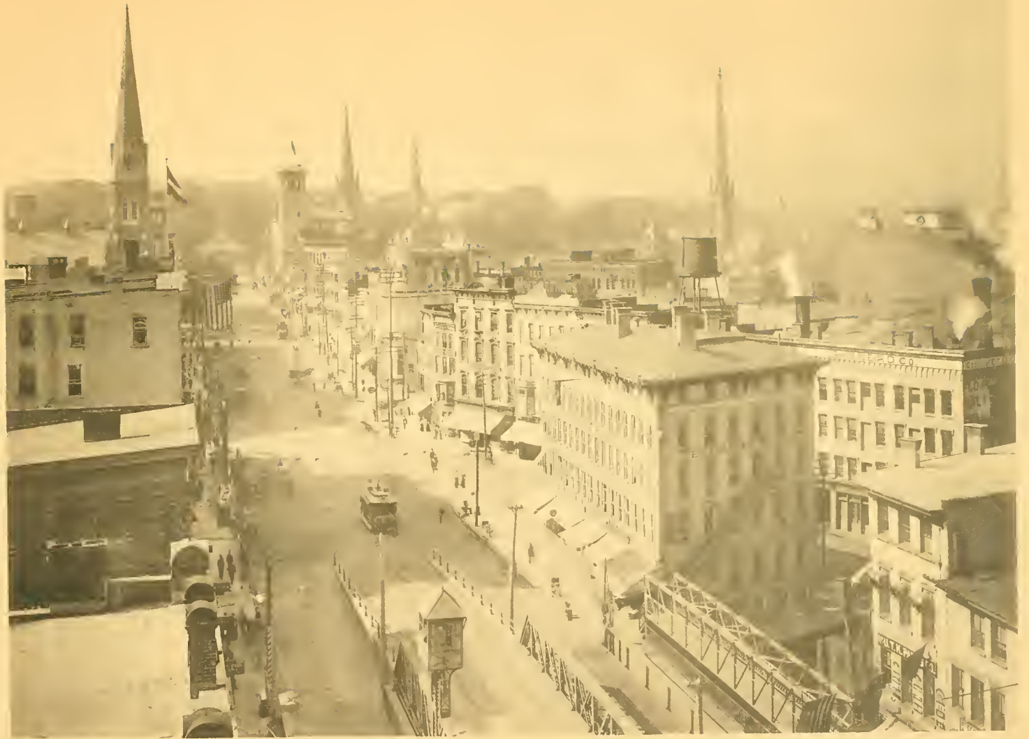
GENESEE STREET, LOOKING UP FROM MARTIN BUILDING.
